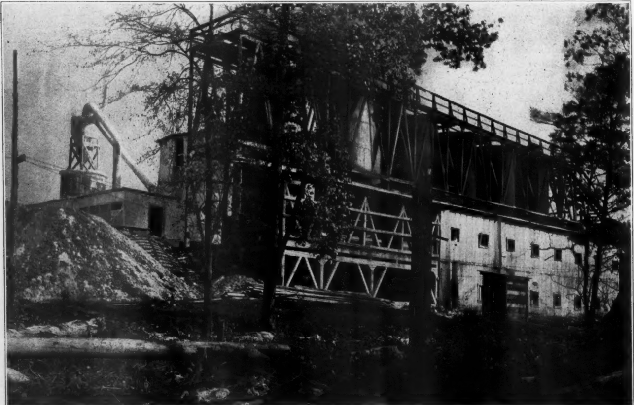
New Kiln Construction
